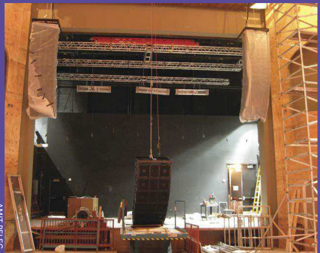
The theatre interior before renovation, above. Below, after extensive renovations, the JBL gear could be flown. Construction was still underway, so the crew used coverings to protect against dust.
